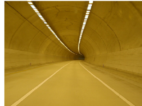
Fig. 1. Tunnels (Kyunggi-do, South Korea).
