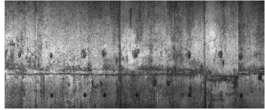
Fig. 17. Image of subway inner wall.
