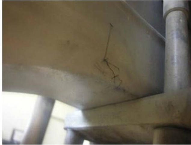
Fig. 4. Fatigue crack on the lower half of a test sample.
